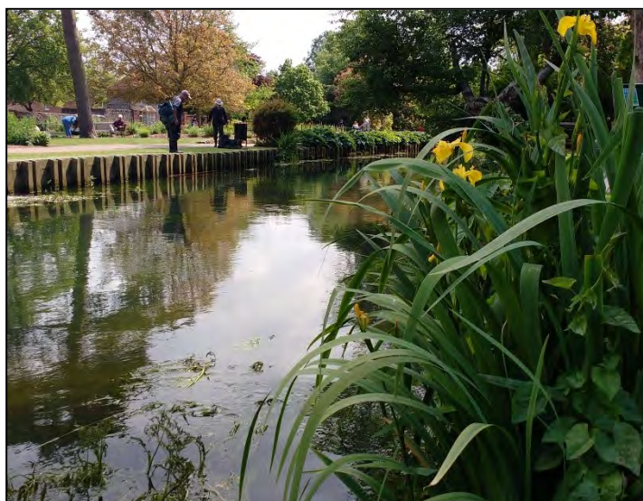
Planting pockets along the edge of a river revetment , Westgate Gardens Canterbury, Kentish Stour Countryside Project
